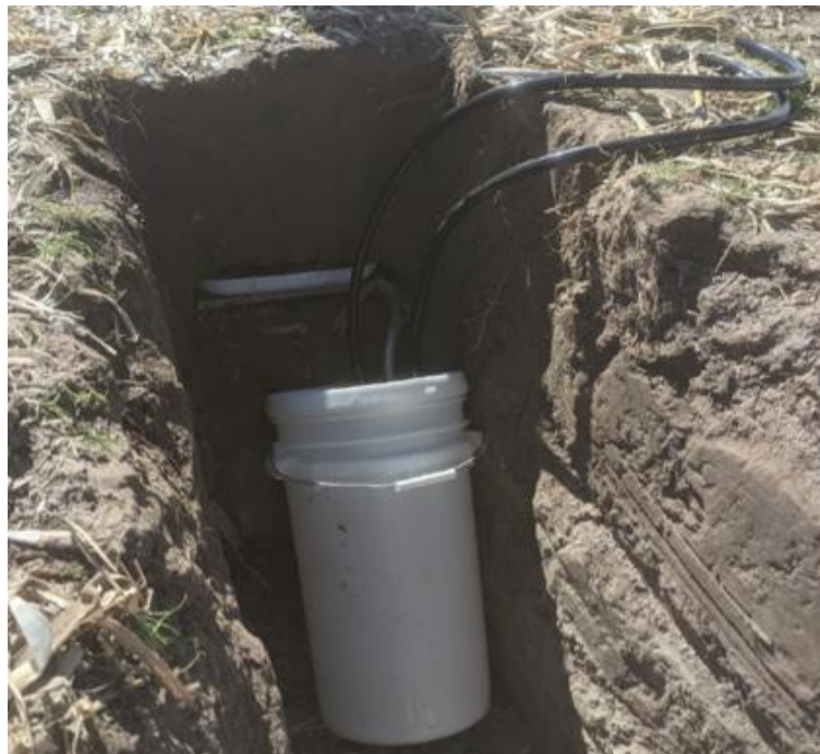
Fig. 2.5. Complete pan lysimeter installation before backfilling with soil.
