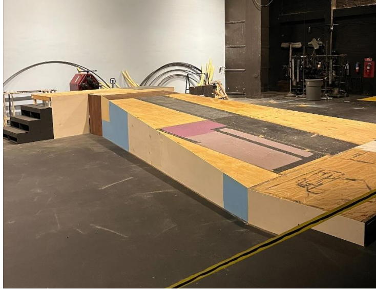
Figure 3.6 – The rake before paints and skinning the top with Eucaboard – Property of author
