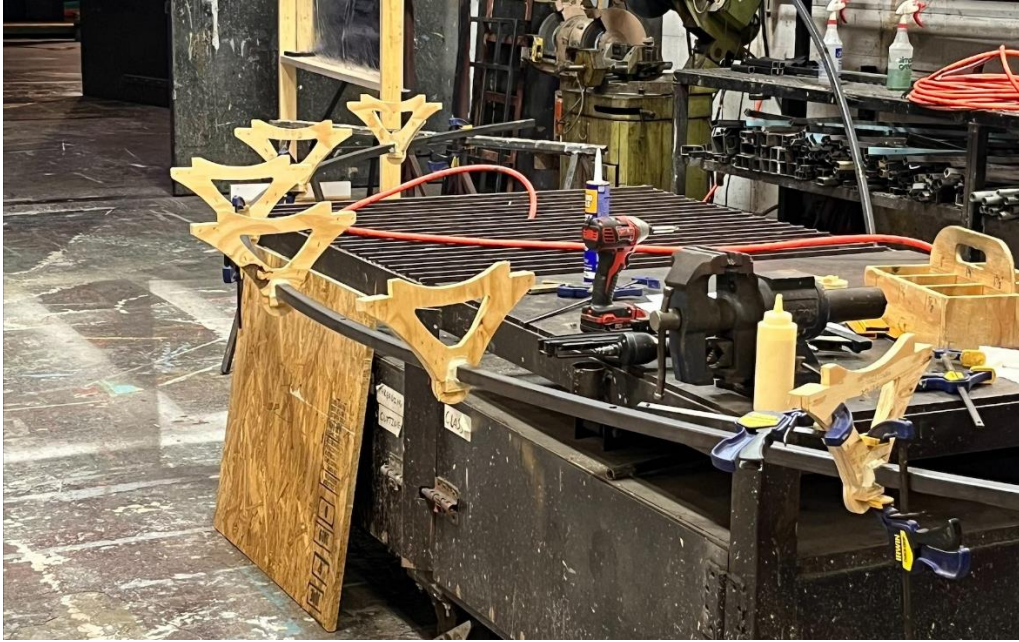
Figure 3.7 – “Vertebrae” attachment to steel with construction adhesive – Property of author.
