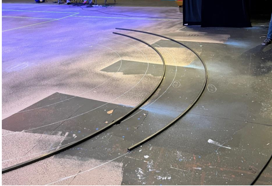
Figure 3.2 – Roller bent steel with scribed radius lines on the stage floor. – Property of author
