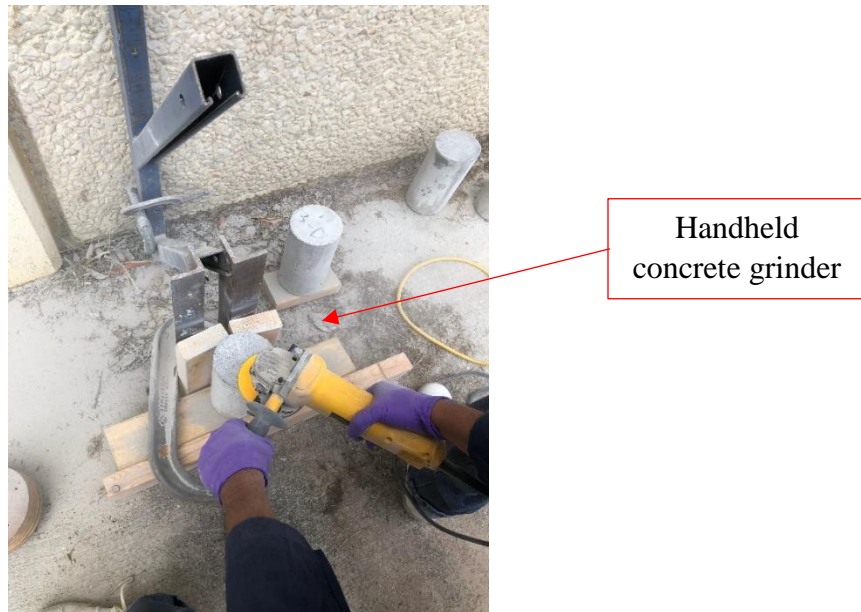
Figure 18. Grinding concrete surface using a hand held concrete grinder
