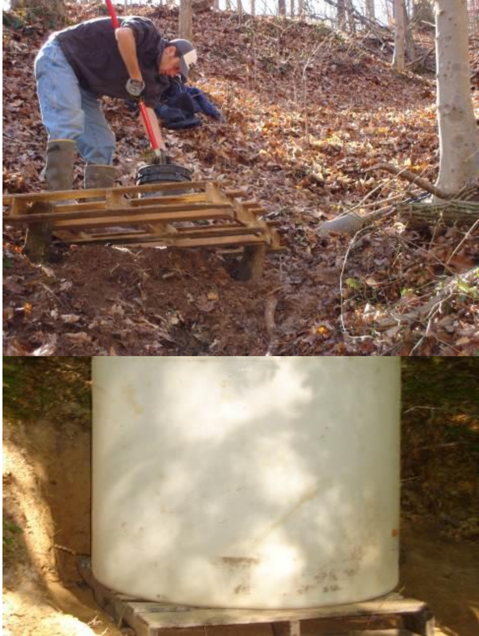
Photograph 3-6. Installation on level tank platform and on leveled earthen surface.
