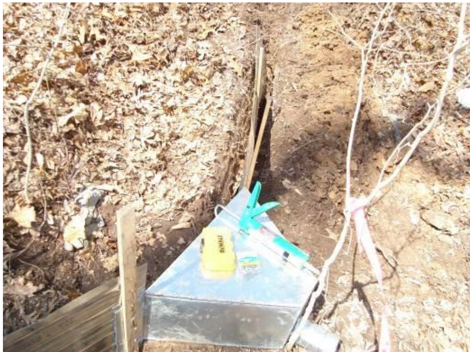
Photograph 3-3. Installation of galvanized metal flume.
