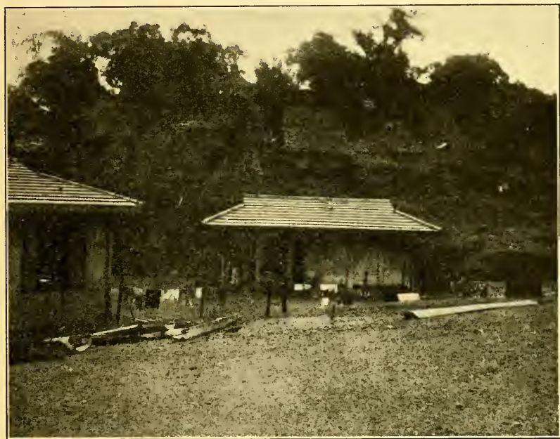
CONCRETE KITCHEN AND LAVATORY BUILDINGS AND NATIVE RESIDENCES.
