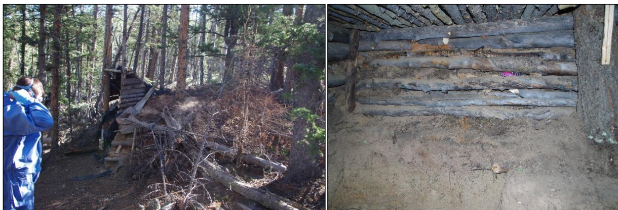
Figure 7-14: Left - Exterior of partially subterranean, hand-hewn log structure. Note the entrance (photo left), and the earthen mound occluding the structure's visibility (photo right). Right - Interior backwall of the structure (following removal of personal items and items of evidence), note hand-hewn log ceiling and wall with subterranean, hand excavated extension. Personal protective equipment was donned due to the volume of rodent scat.
