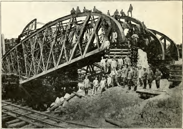
A BRIDGE IN GALICIA BLOWN UP BY THE RETREATING RUSSIANS, BEING INSPECTED BY GERMAN ENGINEERS WITH A VIEW TO RECONSTRUCTION.
