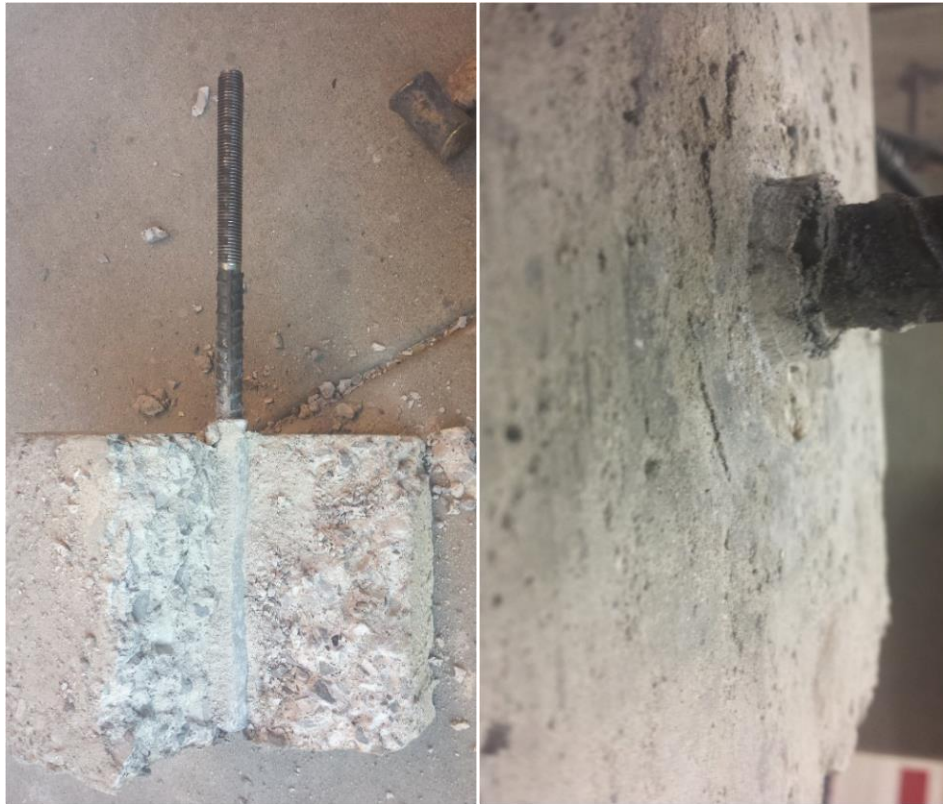
Figure 59: Failure of resin-grout interface.
