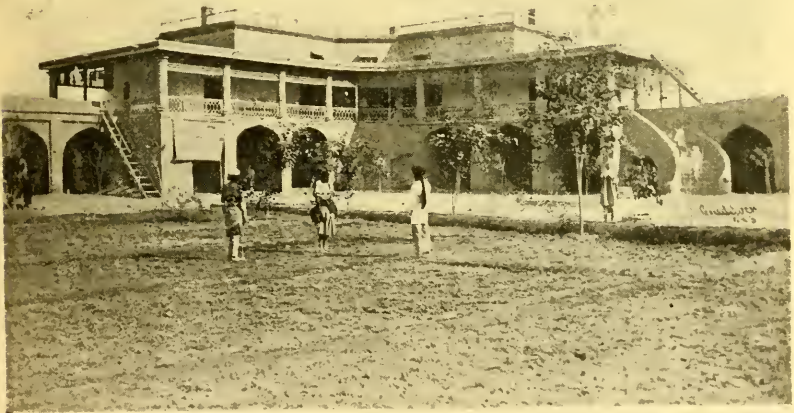
THE MISSION HOUSE ERECTED ON THE OLD WALLS OF THE GURKHATRI.
