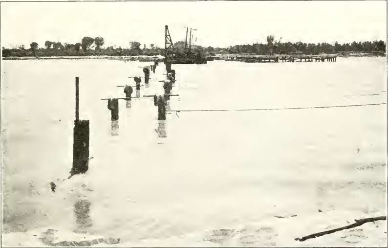
PILING FOR THE RAILROAD TRACK. (Photograph by W. J. Lubken.)
