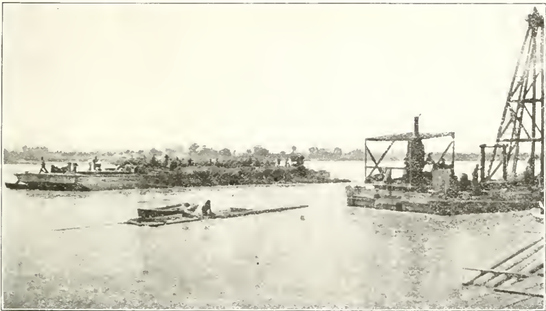
WEAVING FASCINE MATS.
