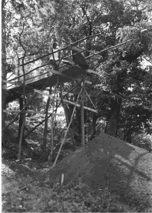
Figure 20: “Use and construction of high wheel-barrow ramp for carrying dirt from top of the high conical mound, Mx o 7” (Mx1078:1941 photo log). Courtesy, Illinois State Museum.
