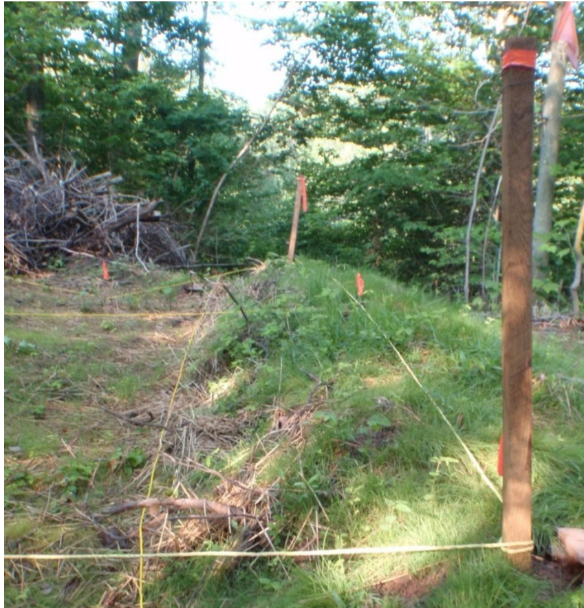
Figure 12. Crest and base of water bar delineated for photography.
