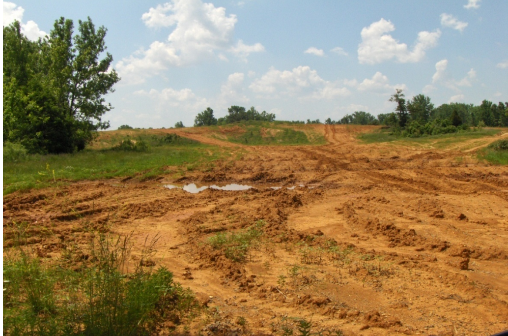
Figure 4. Training area 9, tank trails condition after rain events in the May 2009. Photo taken by Klairoong Pattumma
