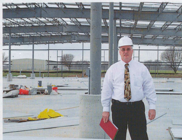
Michael Behrmann stands in what will be the fleet storage building for the University's Transportation Education Center. The program will soon move from its home on the Carterville campus to the 230,000-square-foot complex at Southern Illinois Airport.
