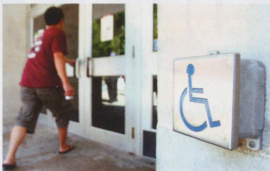
Nearly all entrances to buildings on the SIU campus have wheelchair assisted doors that open from either the outside or inside.
