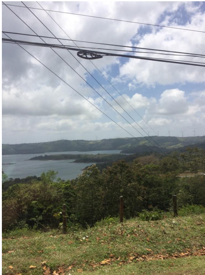
Figure 3: Presa Sangregado Dam and Wind Farm (Smith, 2018).
