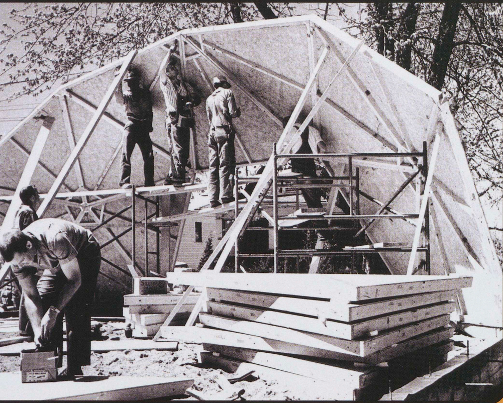
Erected in hours, the dome was built by local contractors and the “spontaneous cooperation” that Fuller advocated.
