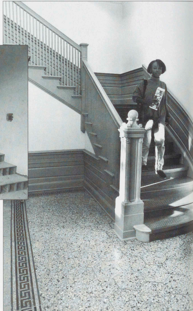
Above: Under construction is the new stairway to the third floor, designed to match the original stairway. At right: The terrazzo floor and stairway at the entrance were repaired.
