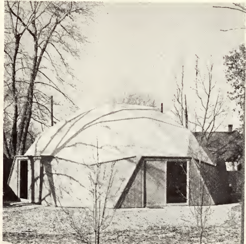
Mr. Fuller's home, a prefabricated geodesic dome, was constructed in Carbondale during 1960.
