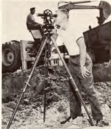
Field work is a major activity in building construction technology.
