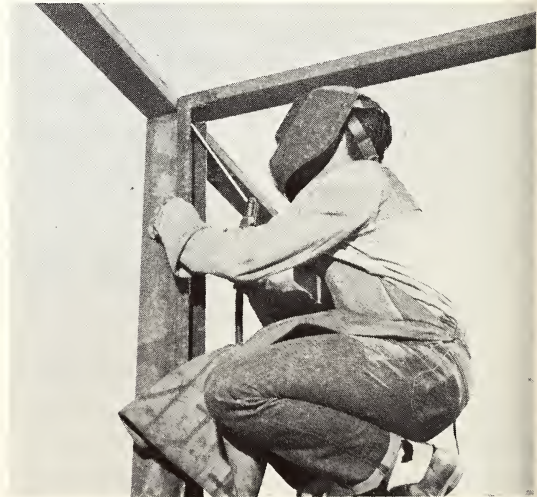
Completing a section of structural steel welding
