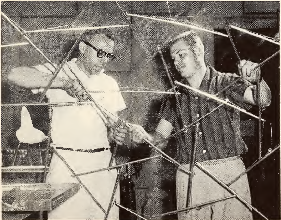
Design students assembling an all-aluminum, continuous-tension sphere which is now on display at the Museum of Modern Art in New York City.
