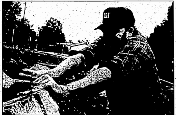
Mack Holderfield of the SIUC grounds crew works to pull rocks from the retaining wall between Mill Street and Lincoln Drive Wednesday morning. This is Holderfield's first year working with the SIUC grounds crew.
