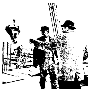
WORKMEN CONFER WHILE CONCRETE IS BEING POURED
