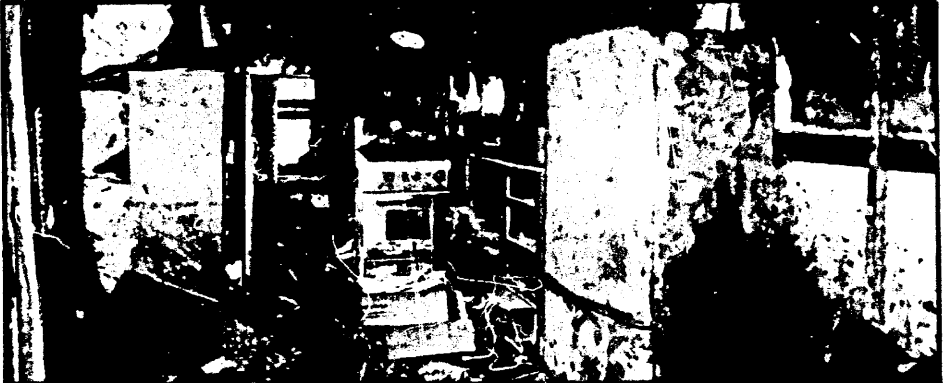
Fire prevention can only help avoid fires such as the one that gutted this Carbondale trailer. Keeping a close eye on wiring and the use of extension cords
