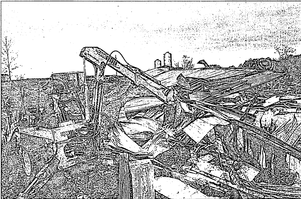
Charlie Hagene, of Elkhart, removes remains of the roof that once stood over his hogs in Elkhart. Hagene has rented this barn from Gene Yates for around 8 years, but the storm that hit southern Illinois Wednesday afternoon destroyed the barn.
