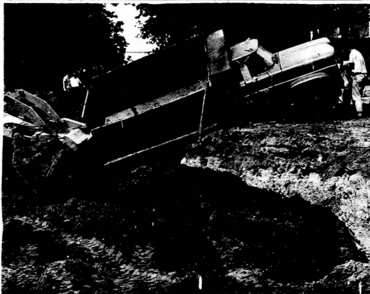
WHOOOPS! —A large dump truck was backed up to this excavation and accidentally overturned Friday afternoon behind Lawson Hall. William Wheately of Wheately Construction Co., Inc.,
