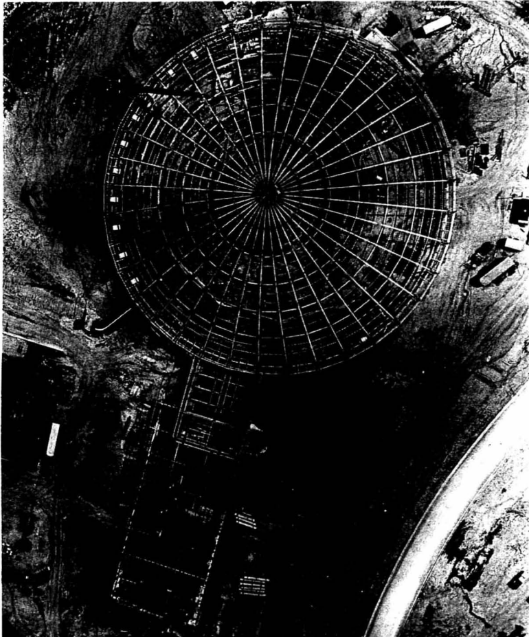
CAGEY CONSTRUCTION - This aerial view of the new Physical Education-Military Training building framework makes it appear to be a giant bird cage with a handle. The building will probably not be completed until next year because of work stoppages caused by bad weather and a carpenter's walkout. (Photo by Hal Stoelzle)
