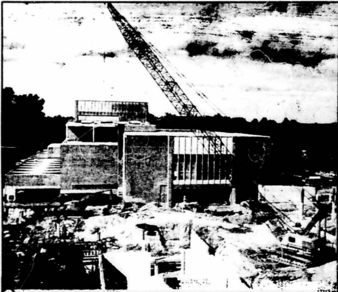
Student Center under construction in 1969.
