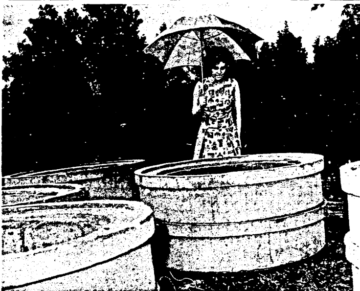
MORE PHONES FOR SIU - Concrete conduit pipes, each containing 12 smaller conduits 3/4 inches in diameter, are being installed by the General Telephone Co. along University Avenue. The 2,100 pairs of lines to be carried in the con-
