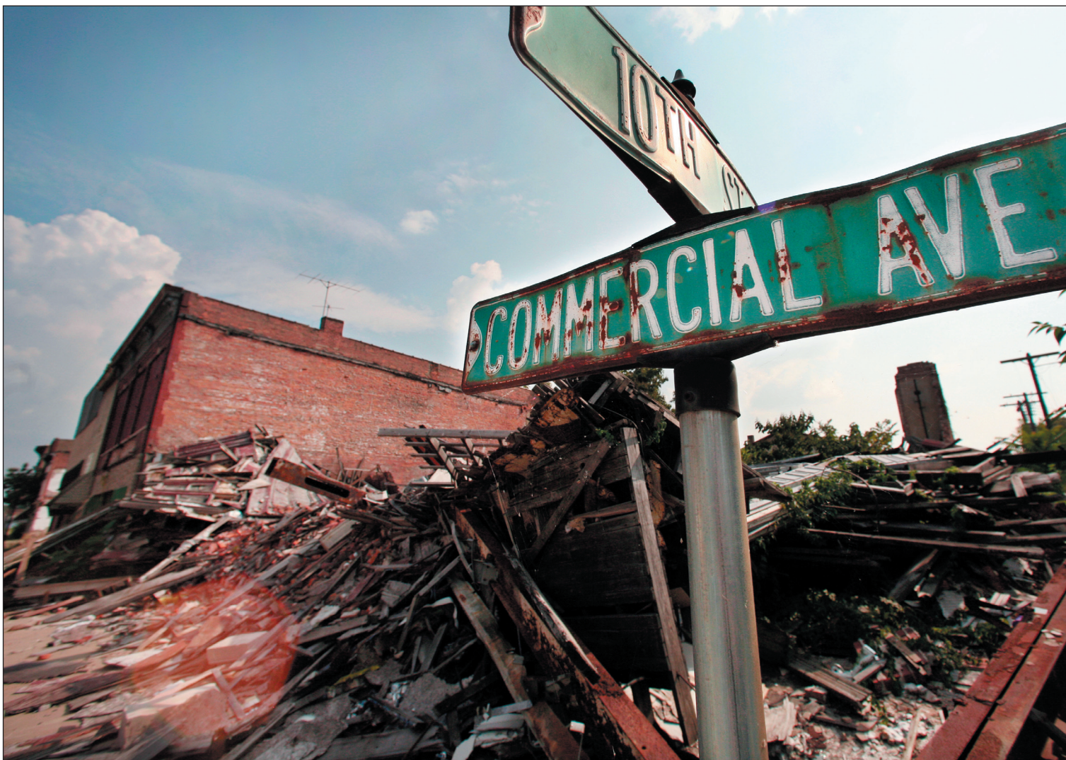
The remains of a building spill onto the sidewalk at the corner of 10th Street and Commercial Avenue in Cairo. The city of Cairo has seen a dramatic decline in population in the past 80 years. About 34 percent of the citizens live below the poverty level. But university groups and
