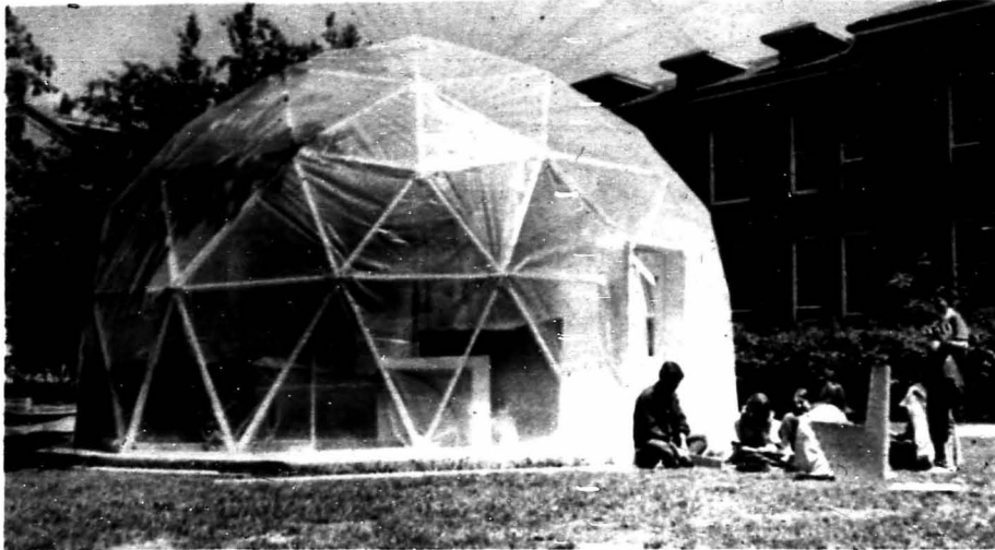
No, it's not a new classroom building. The portable dome located west of the Allyn Building is the center of information and resources for Alternative 71. The structure, which is 16 feet high and 40 feet in diameter, was built by Tony Pugh, lecturer in the design department, and a team of students. Plans are to keep the dome for possible later use. Total costs of the facility, including utilities, is $1,500. (Photo by Fred Pfeifer)
