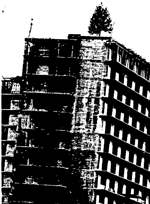
HO, HO, HO - The jolly workers on the new University Park 17-story residence hall got into the spirit of Christmas and hiked a tree to the top of the building, after a casual suggestion from William A. Volk, associate University architect. Some students added a festive touch with a robe of bathroom tissue.
