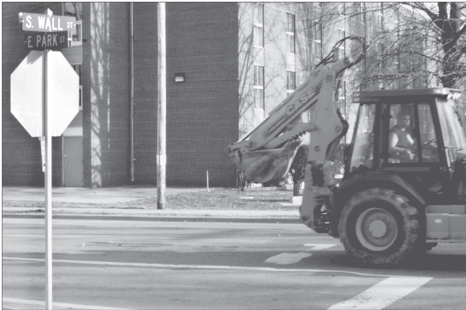
A Backhoe operator stops and prepares to turn left onto South Wall Street. There are plans in place to begin repaving Wall Street from East Park Street to Mill Street.
