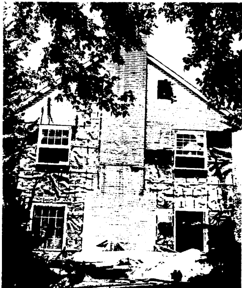
RAZING CONTINUES - The work of razing buildings south of the University Center is progressing. The buildings are being removed to make way for new construction. This was the Talbot Abbott house purchased by the University for $68,000 and sold for less than $1,000 in order to clear the site. Abbott was formerly dean of the College of Liberal Arts and Sciences.
