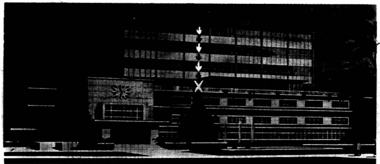
DOTTED LINE INDICATES 56 FOOT FALL BY CONSTRUCTION WORKER
