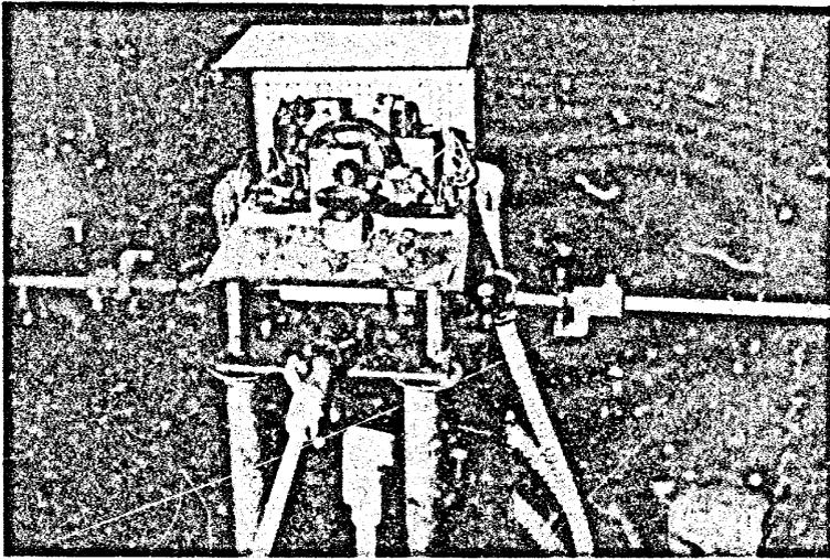
The iron innards (above) of Pulliam Hall's four-faced clock keep the time with help from protruding shaft rods, one for each face. At left, Physical Plant workers spruce up the
