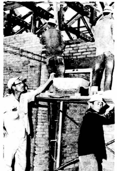
U.S. ENGINEER SUPERVISES WORK ON HOSPITAL FACILITY
