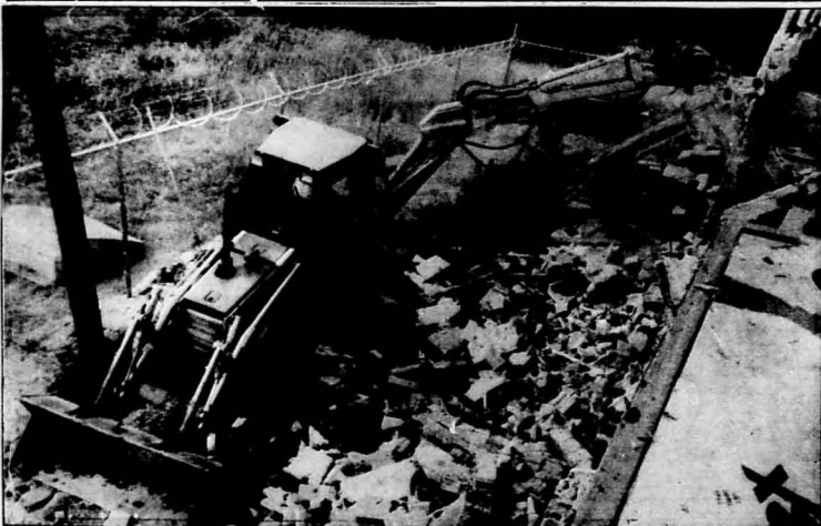
A backhoe with a hydraulic hammer from Morgan Construction in Murphysboro, breaks down the east wall of the Jackson
