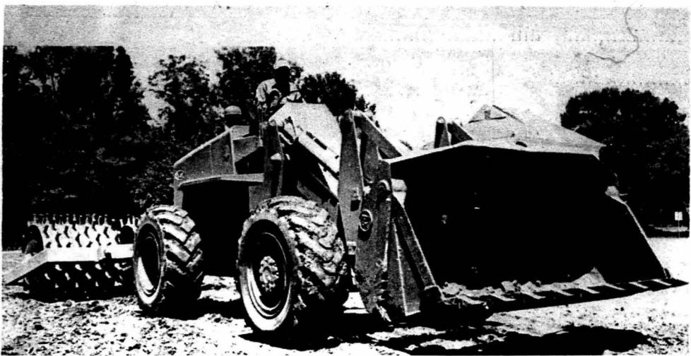
Doyle Smith of R.B. Stephens Construction drives earthmover Tuesday at Lot 107.
