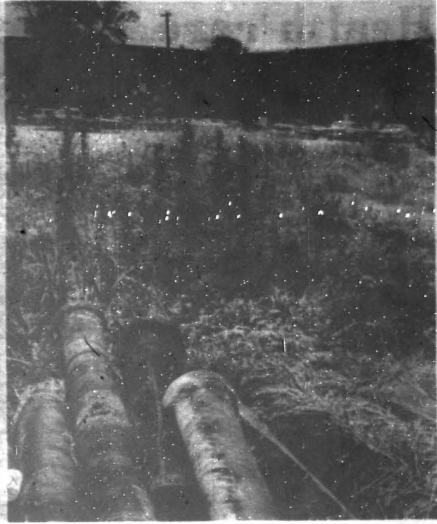
These cast-away pipes on city owned lot near Wilson Hall impede mowing and give rats a place to hide.
