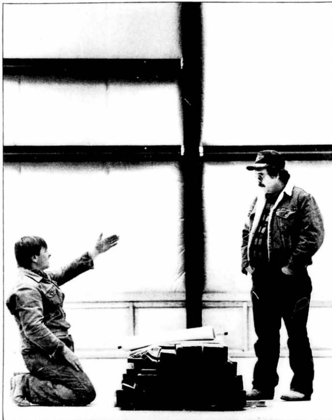
Morgan Construction foreman Bob Roncey of Marion, left, discusses plans for completing the Library Storage Facility on
