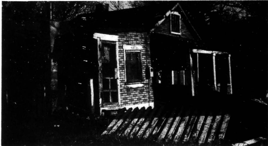
A sagging porch, broken down fence and tar paper roof characterize this house located on North Washington Street in the Northeast section of Carbondale. This area contains
