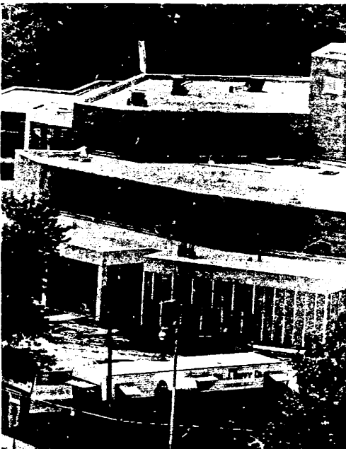
READY BY FALL —The new $3,266,109 Classroom Building Group, photographed from Morris Library, will be in use in September, University officials report. (Photo by Hal Stoelzle)
