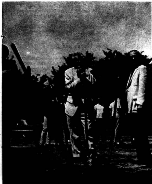
GROUND BREAKING - President Delyte W. Morris (center) leans on a shovel handle and joins with SIU Board Member Harold R. Fischer (right) in beaming approval as ground was broken last week for the $10.5 million University Park dormitory project. They were probably envisioning the completed 17-story women's dormi-
