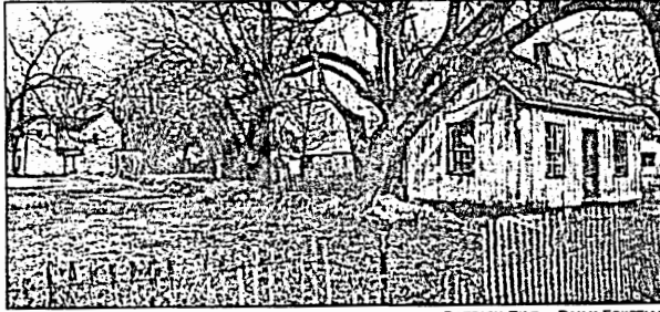
The Samuel Dalton house located behind the John A. Logan House and Museum in Murphysboro was purchased from Logan in 1887. Dalton born a slave at age 24 enlisted in the Union Mississippi Fleet during the civil war.
