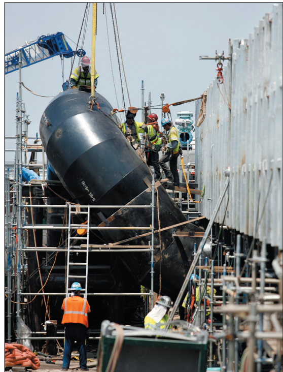
Construction workers install large water pumps along the 17th Street Canal in New Orleans, Louisiana in an effort to help prevent flooding during future storms, Aug. 8. Residents of New Orleans are still working to recover and rebuild their city two years after Hurricane Katrina hit the coast with devastating force and flooding.
