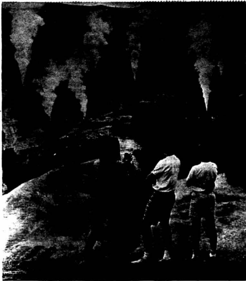
NATURE'S TEAKETTLES —Tourists watch a well cleaning operation at the Geysers in Sonoma County, Calif. Five of these wells will carry 550,000 pounds of steam per hour to a new generating unit of Pacific Gas and Electric Company's Geysers Power Plant. It is the only electric generation installation in North America using geothermal steam to power turbine-generators on a commercial basis. The wells are from 500 to 5,000 feet deep. (AP Photo)
