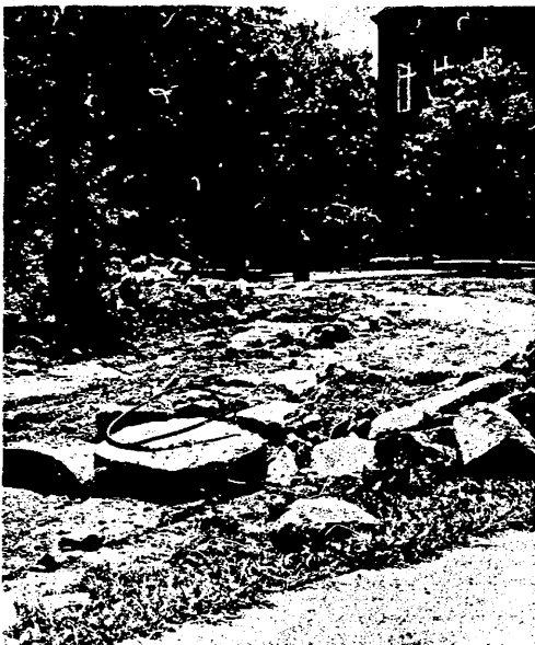
CRACKING UP — That term would adequately describe the condition of this road, located between Old Main and the gymnasium. Physical plant workmen are cracking and removing a section of this paved road. The roadbed will eventually be sodded in and then made into an uninterrupted expanse of campus.
