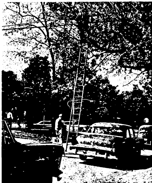
TRAFFIC ISLAND - Art Boatright watches as Bill Morris stands on a ladder in the middle Grand Avenue to trim branches around utility lines. The work, done Friday afternoon, was near Illinois and Grand Avenues.
