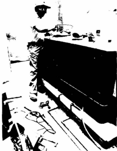
The new gym will be equipped with a diesel generator, as Jerry Millette of Presley Plumbing and Heating of Paducah, Kentucky, prepares the fuel line.
